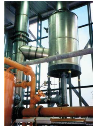
Installation of a DC-2-300 SUPERMIZER servicing a 300 HP. Fulton Hot Oil Boiler. Note simple support frame eliminates structural roof support members
