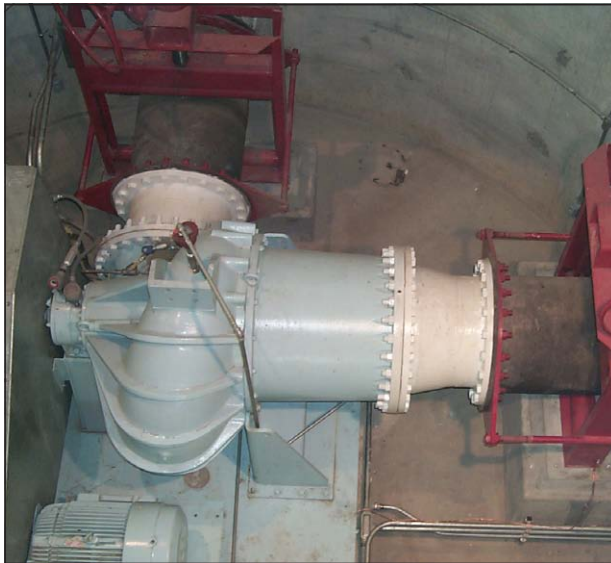
Pump installation at California Irrigation District.
